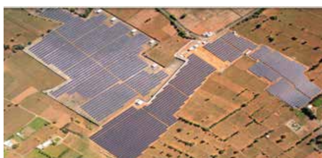
Erode District, Tamilnadu - Total SPV Capacity: 16 MW
