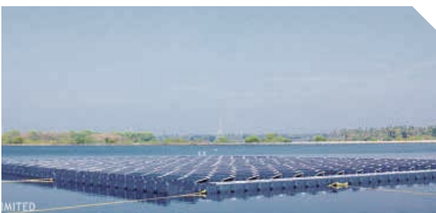
India's First Floating Solar Plant, Kerala - SPV Capacity: 100 kWp
