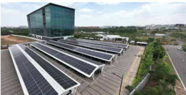
Coimbatore, Tamil Nadu - Rooftop Car parking, SPV Capacity: 626 kWp
