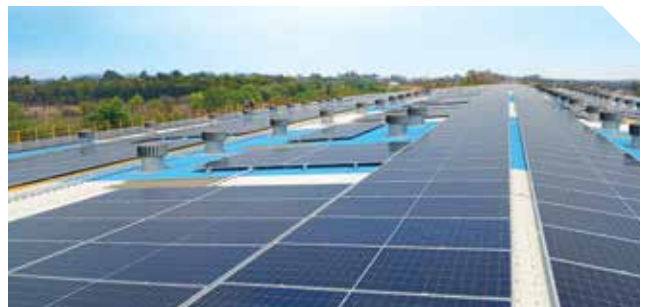
Coimbatore, Tamil Nadu - SPV Capacity: 1 MW
